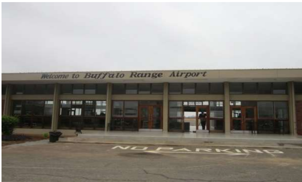
Figure 3-6: Buffalo Range Airport Passenger Terminal Building
