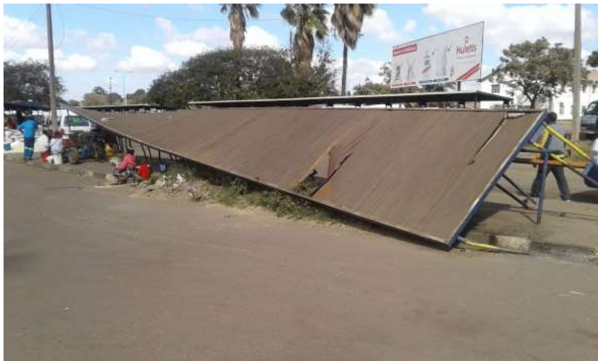
Figure 2-24: A Fallen Bus Shed at a Taxi Rank in Harare
